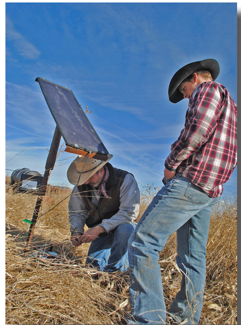
Ranchers set up a photovoltaic panel and a battery back-up to electrify a fence after moving cattle to a field in Kansas. Mike Breen Photo
