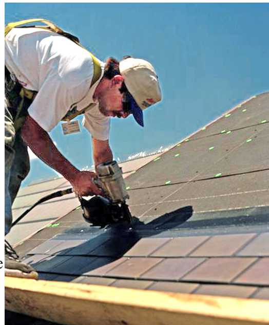
Installation of Photovoltaic shingles. DOE/NREL - Warren Gretz Photo
