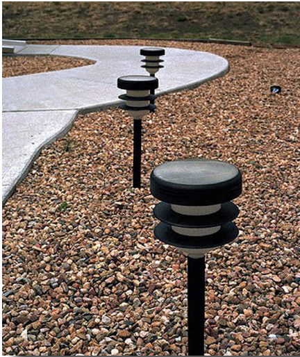
Photovoltaic Walkway Lights DOE/NREL - Warren Gretz Photo
