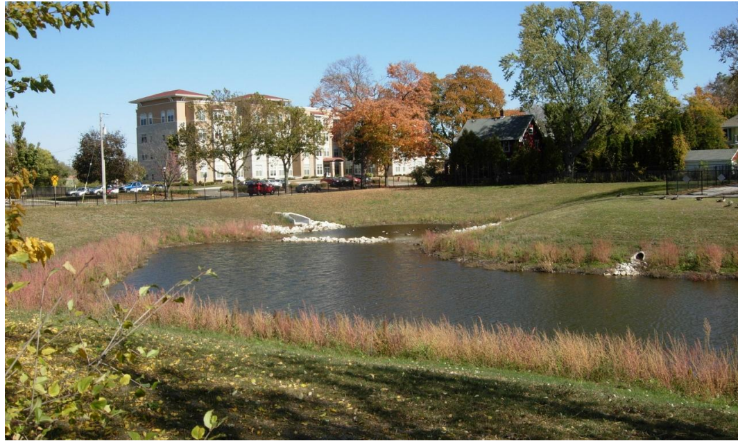
Stormwater retention pond in Waukesha, Wisconsin. The pond was constructed in 2011. Nine single-family homes were purchased by the city, residents relocated, the homes demolished, and the pond constructed. The area was subject to repeated severe stormwater flooding. Image by Aaron Volkering. https://www.flickr.com/photos/87297882@N03/13851531525 CC BY
