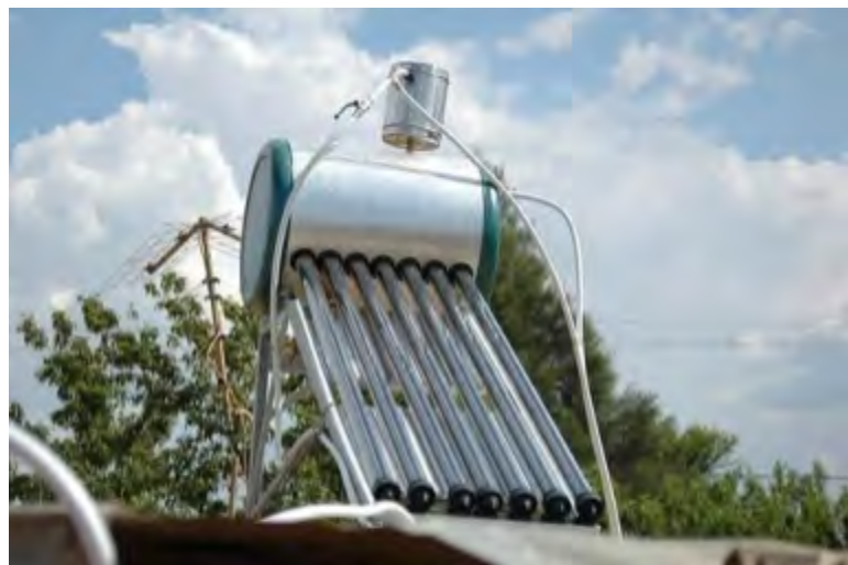
A solar water heater on the roof of a house. The water is in the tank.
