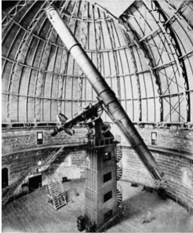
The largest refracting telescope in the world is at the University of Chicago's Yerkes Observatory in Wisconsin and was built in 1897. Its largest lens has a diameter of 102 cm.
