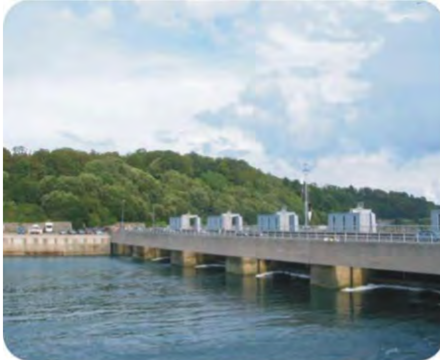
Rance tidal power plant by Dani 7C3, https://en.wikipedia.org/wiki/File:Rance_tidal_power_plant.JPG CC BY-SA
