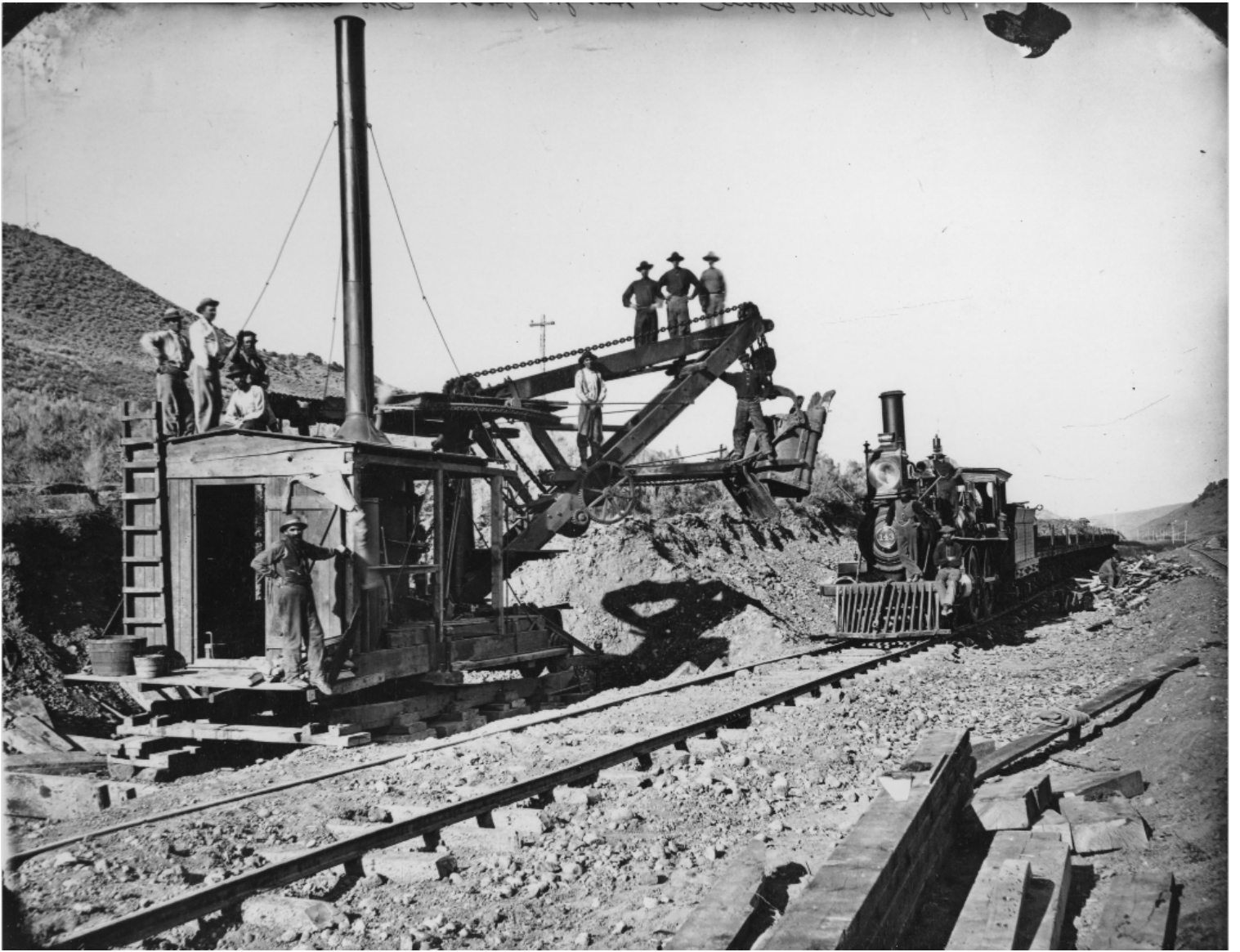
Steam shovel at Hanging Rock. No. 143 hauling broken rock to fill in around ties and to widen embankments. Photo by A.J. Russell. Digital Image © 2008 Utah State Historical Society. All Rights Reserved.
