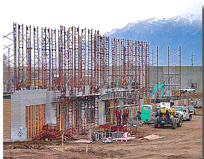
Scaffolding is set in place to lay cinder block during this commercial construction project in Riverdale, Utah.
