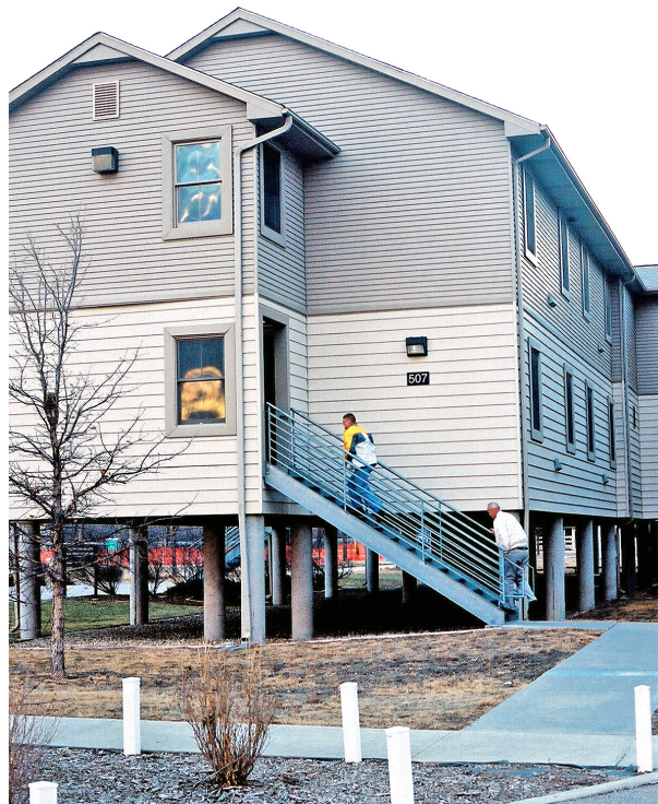
A building in a flood plain is built on pillars. Camp Ashland, Nebraska Mike Breen Photo
